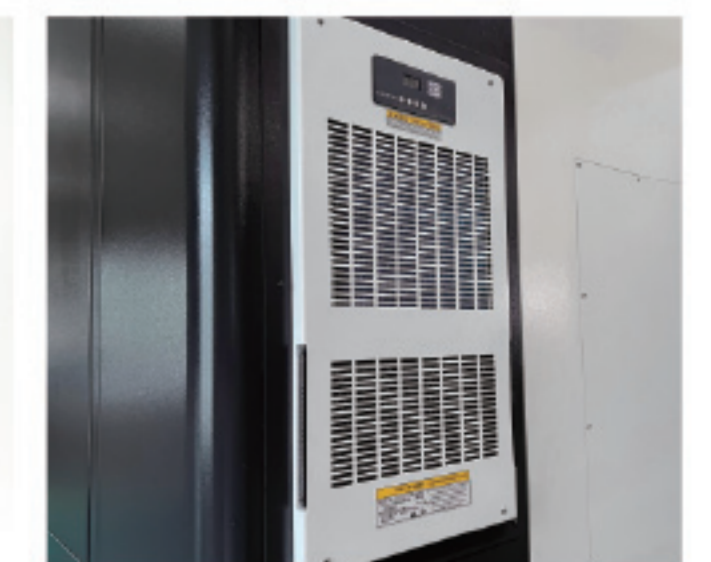
Electric cabinet air conditioner
